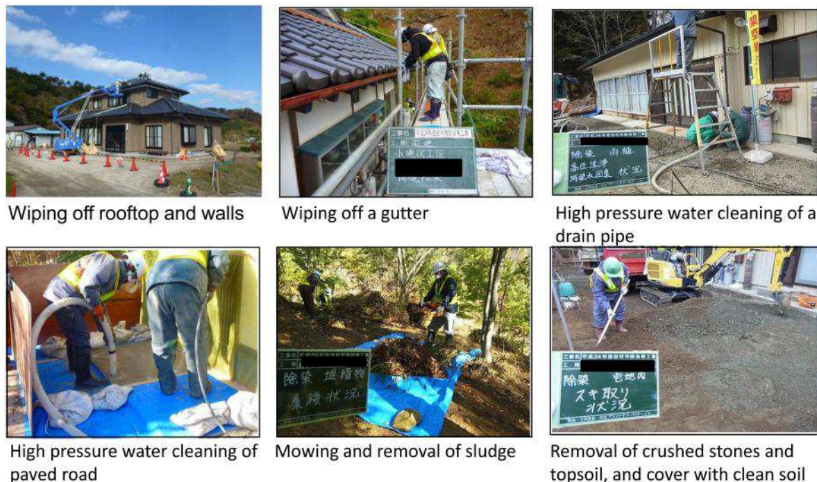
Figure 4: Demonstration of some decontamination methods utilized in the remediation works.
